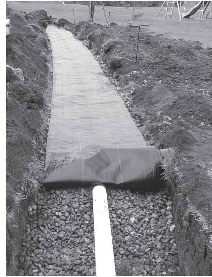
Figure 13. Gravel-filled trench covered with geotextile fabric.
